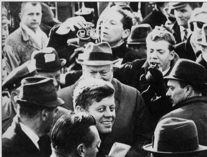
ABOVE LEFT President John F. Kennedy arriving at the groundbreaking ceremony for the Federal Pavilion, December 14, 1962. World's Fair Corporation photograph; Peter M. Warner Collection.
