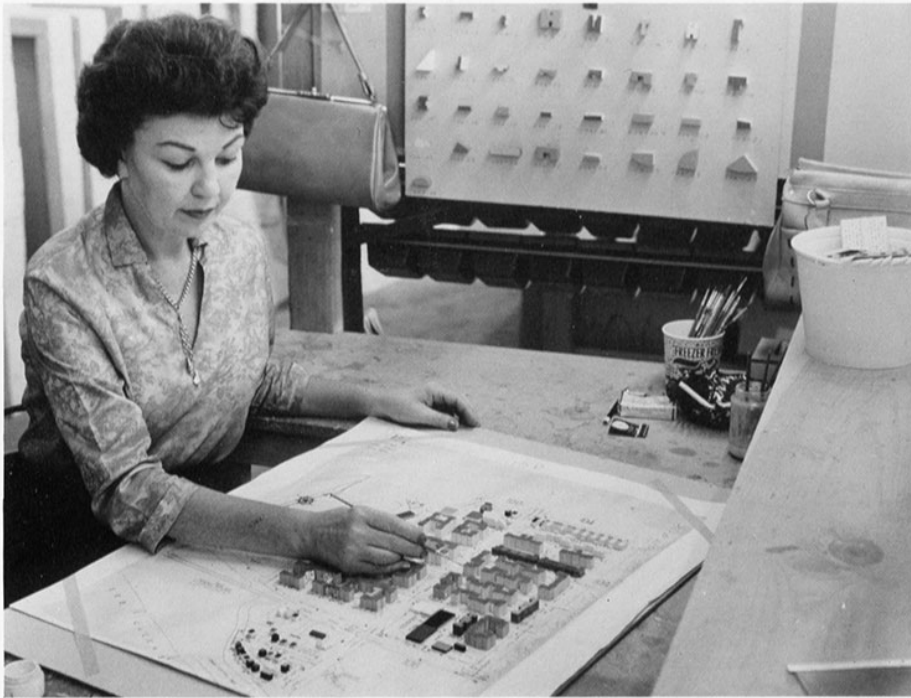
ABOVE: Worker placing building models on a section of the Panorama, 1963.
