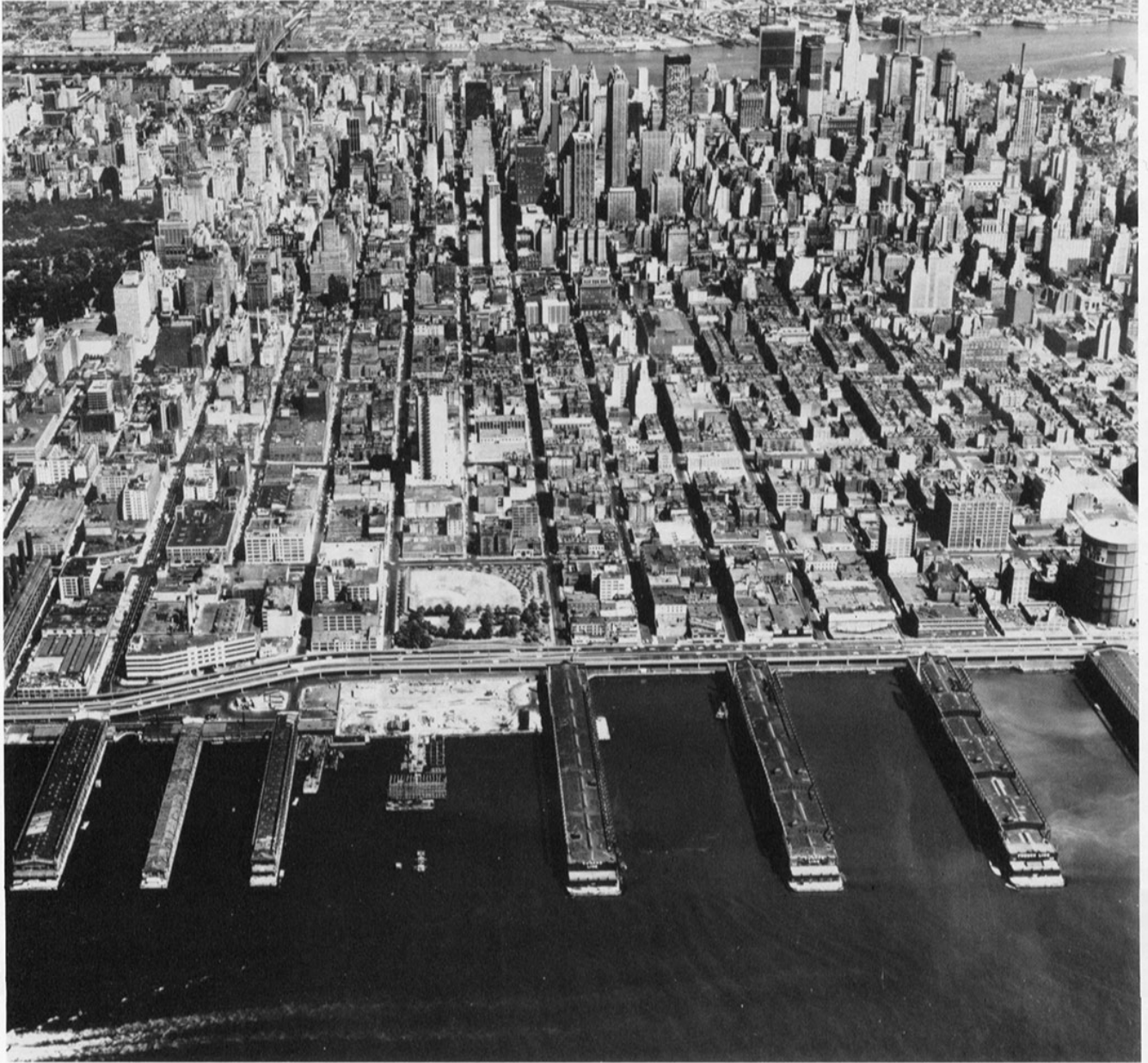
Aerial photograph by Aero Service Corporation showing the west side of midtown Manhattan (used during the construction of the Panorama), c. 1961.
