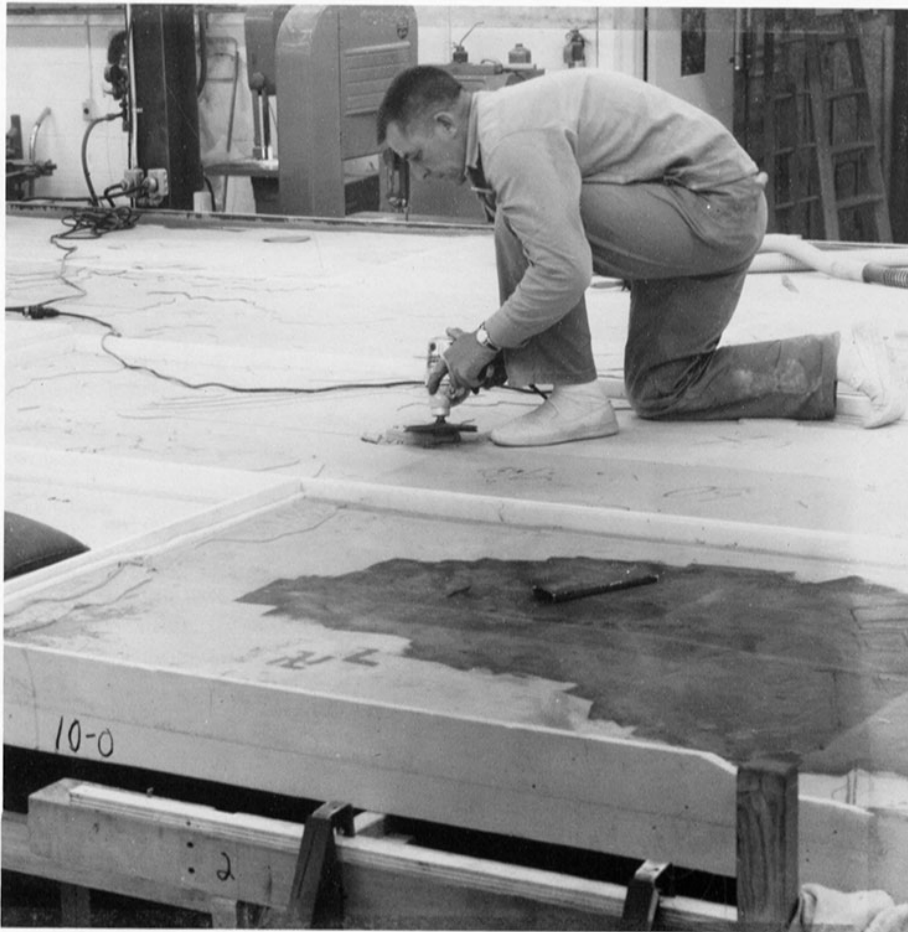
Worker sanding elevation contour on the Panorama, 1963.
